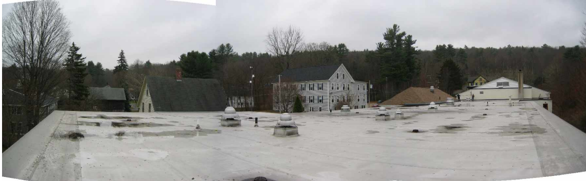
PHOTO 1 - FLAT ROOF - NOTE NO PATTERN OF PONDING
