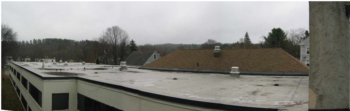
PHOTO 3- FLAT ROOF - NOTE NO PATTERN OF PONDING
