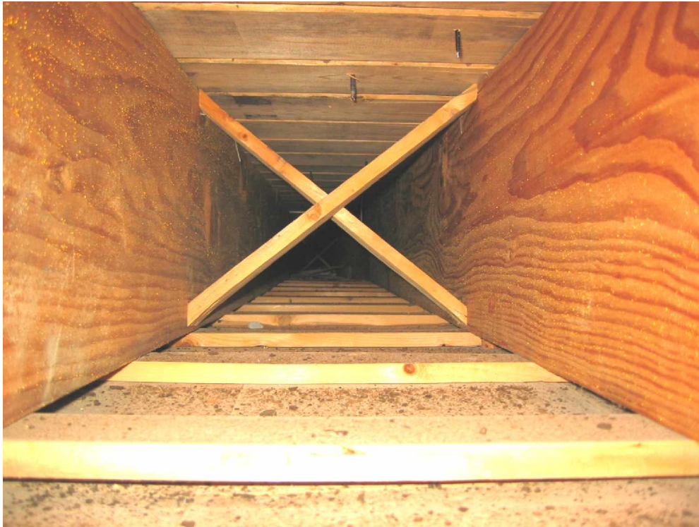
PHOTO 4 - TYPICAL VIEW OF 1-1/2 x 13 RAFTERS LOOKING FROM OBSERVATION OPENING DOWN THE BAY (Room 207)
