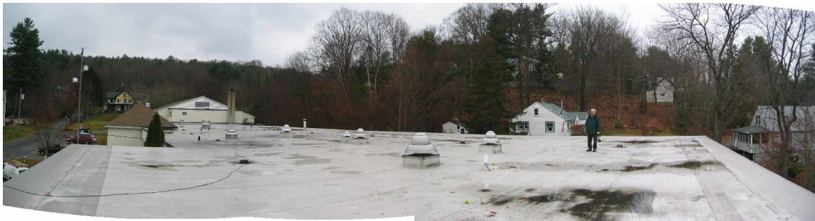
PHOTO 2 - FLAT ROOF - NOTE NO PATTERN OF PONDING
