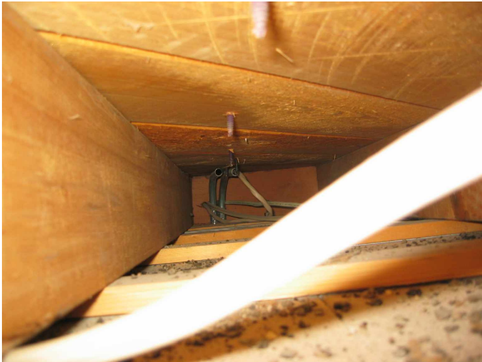
PHOTO 15 - VIEW OF RAFTER BAY IN HALLWAY
