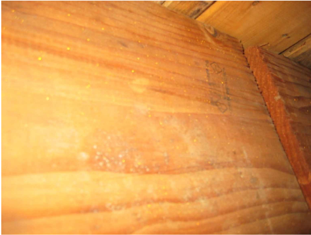
PHOTO 8 - TYPICAL END CONFIGURATION OF 1-1/2" x 13" RAFTERS
