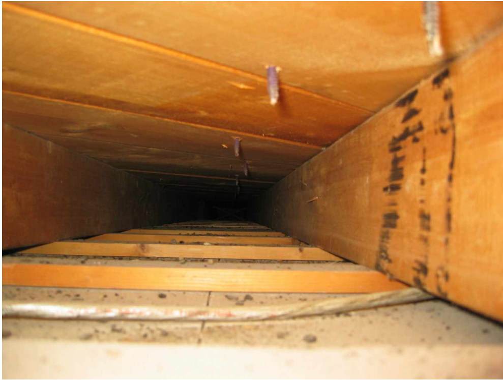
PHOTO 14 - VIEW OF RAFTER BAY IN HALLWAY
